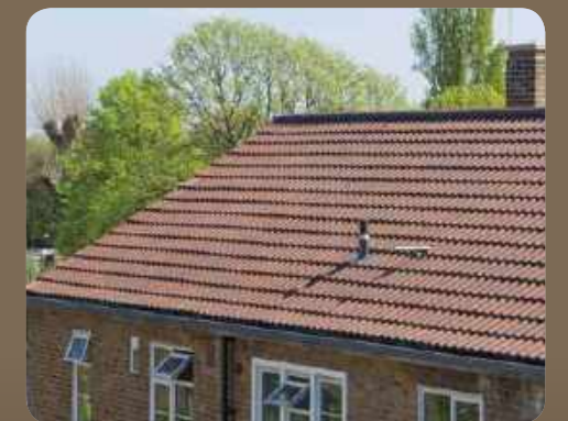
Landmark Double Roman, Brown Brindle, Hackney Homes, Hill Court Estate, Hackney, London
