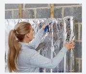
4. Tape and seal the perimeter and overlaps using YBS Aluminium Foil Tape, creating an airtight vapour control barrier.
