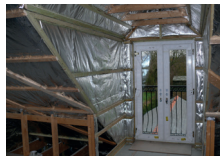
YBS SuperQuilt being installed in a dormer
