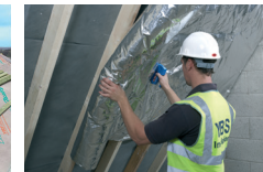
YBS SuperQuilt being installed under rafter
