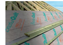
YBS BreatherQuilt being installed over rafter
