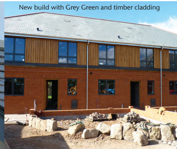
Grey green on gable roof with block end capped ridge.
