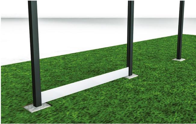
**1** When using the slot between method, Fence Panels need to be cut into 1.8m lengths. Posts must be 1.8m apart and include an extra 5mm gap each end to allow for expansion of the Panels.
