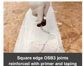
Double reinforced trim joint
