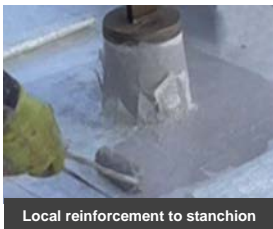
Local reinforcement to stanchion
