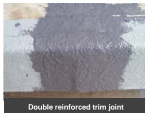
Double reinforced trim joint
