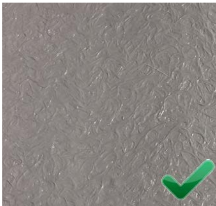
First coat applied at the correct coverage, with the matting fully consolidated and “swirly” in appearance
