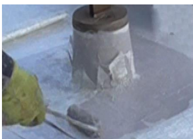
Local reinforcement to stanchion
