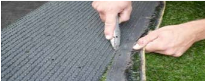
Step 3 – Cut Artificial Grass To Size
