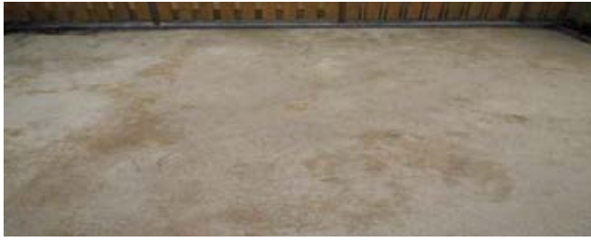
Step 1 – Apply Foundation For Artificial Grass
