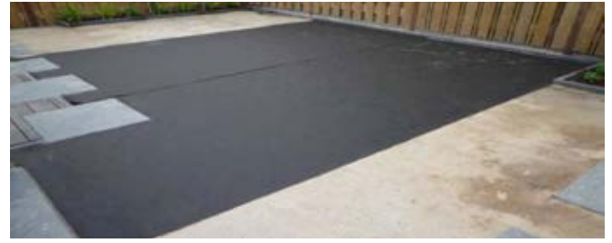
Step 2 – Apply Membrane/Pressure Distribution Cloth
