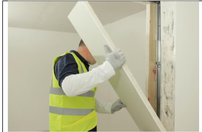
Figure 4 Window reveal installation
