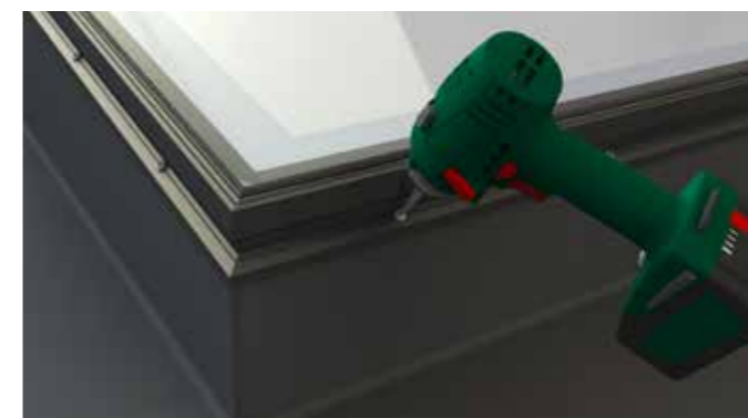
3 Screw the Rooflight onto the kerb using appropriate fixings. Secure it 150mm from the ends and 250mm centres.
