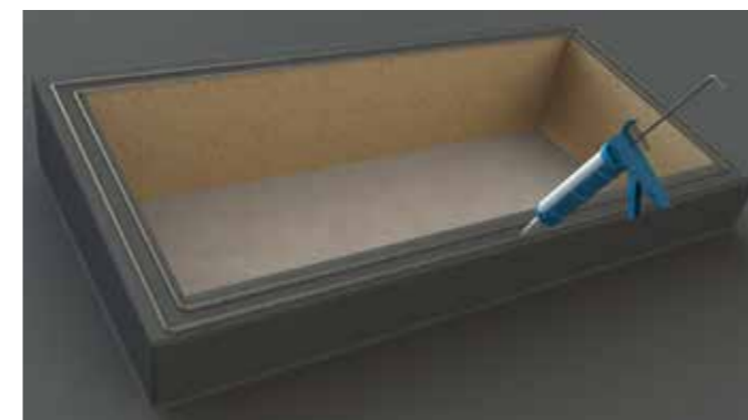
1 Run a continuous bead of sealant around the perimeter of the kerb for the frame to sit on.
