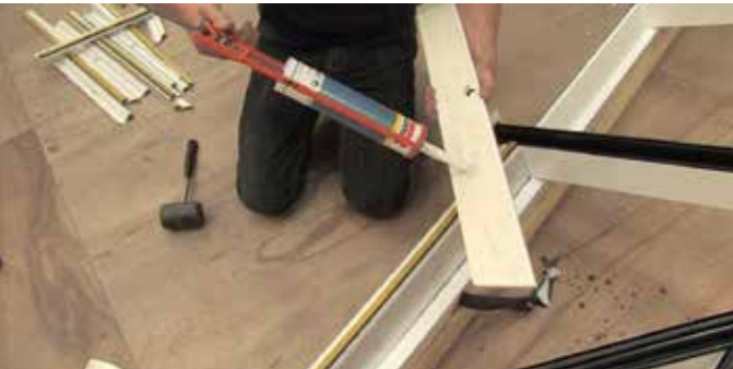
3 Silicone the foam board securely into place.
