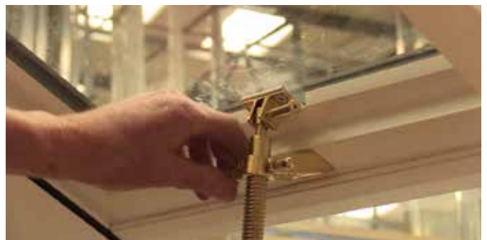
12 Locate the spindle and tighten bolts to secure.
