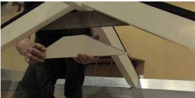
3 Fix the gusset cover over the hidden tie bar. Secure with screw.
