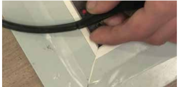
8 Snip the wedge gasket internally at the corners.
