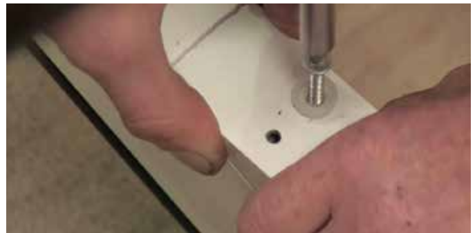
4 Fix the gusset with screws provided and cover with screw caps.
