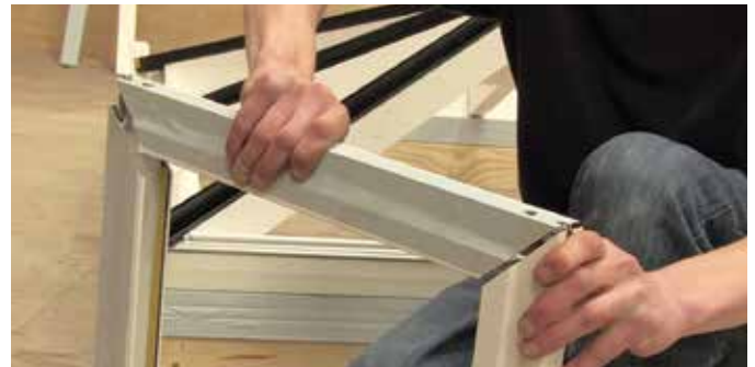
2 Remove one side of the roof vent sash.
