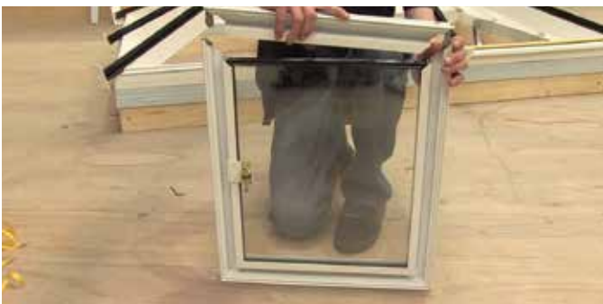
5 Locate the side of roof vent sash by slotting the corner cleats into the adjoining internal chambers.
