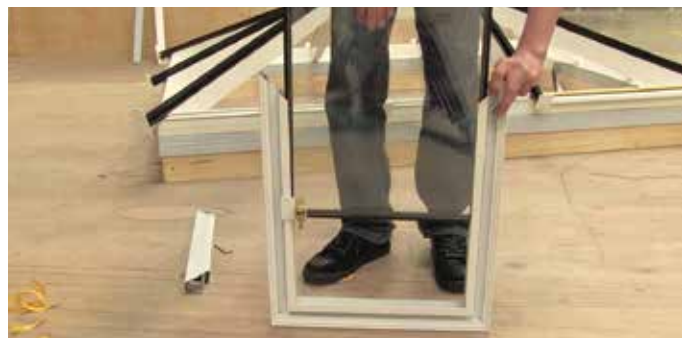
4 Slide glazing into roof vent sash and press down.
