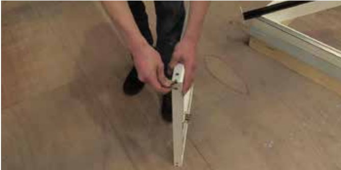
1 Loosen grub screw on sash corners with an allen key prior to glazing roof vent.
