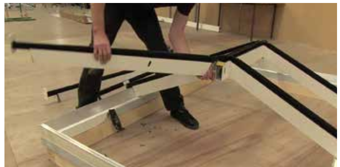
6 Loosen off the top hip bracket screw and position into the slot provided. (See page 6 & 7 for contemporary lantern hip installation)
