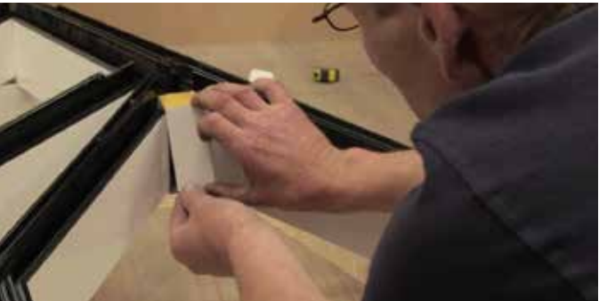
4 Where there is no bell rafter, glue internal ridge end caps onto each end of the ridge.
