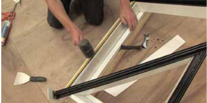
2 Knock down tight with a rubber hammer.
