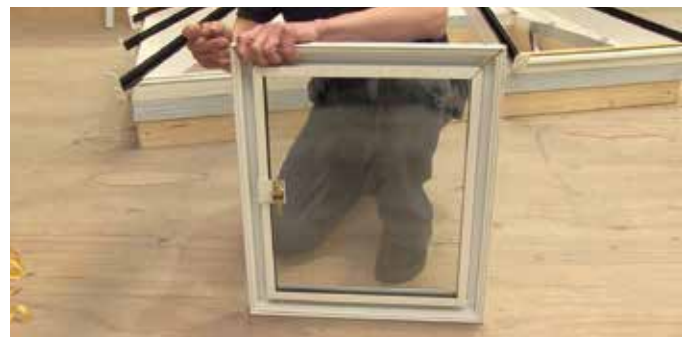
6 Secure the side into place by tightening the grub screw at the corners.
