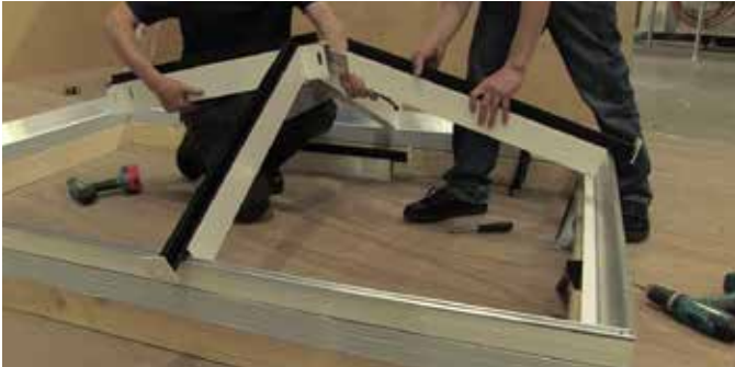
1 Slide the bell rafter over the pre-fixed ridge bracket.
