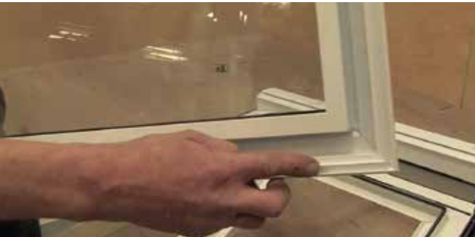
9 When fitting the roof vent sash position the sash into place with the integrated hinge channel.
