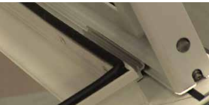
11 The channel locates at approx 70 degrees in the opening position.
