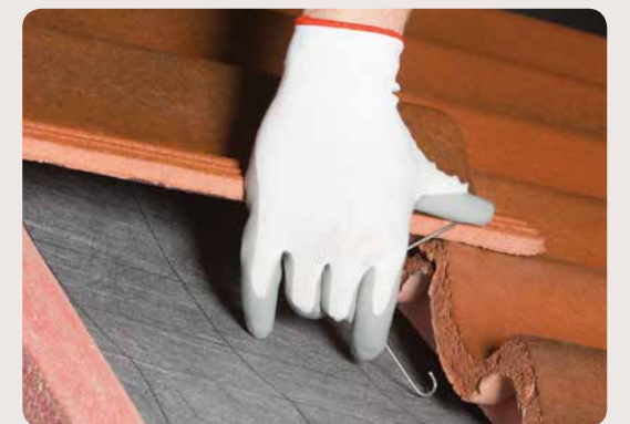
THE MULTI-AWARD WINNING INNOFIX CLIP: A NEW WAY OF TILE FIXING FOR THE INDUSTRY
