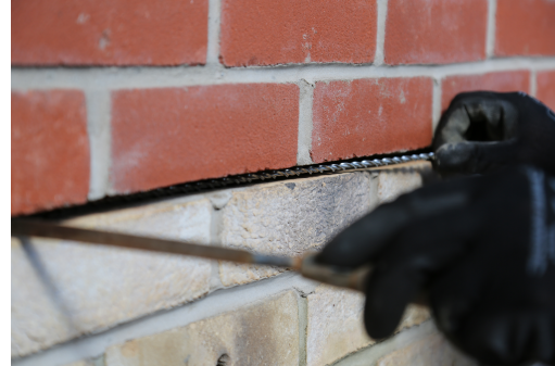
Photo demonstrating helical bar bonding use of Strucsol Grout
