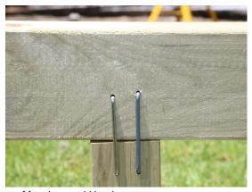
Ordinary pile: 2-s/steel 'U' wire dogs & 2-100x4mm s/steel skew nails (not shown)
