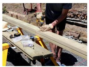
Measure the pile spacings and cut bearers to length, taking care to not have joins on adjacent piles.
