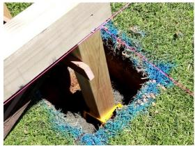
Place bearers on piles and tack in place with skew nails. Straighten bearer lines and prop in place with temporary braces attached to pegs set in the ground.
