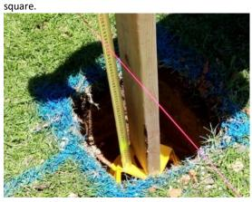
Mark out pile locations & excavate footing holes to correct size & depth.
