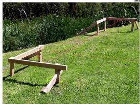
Mark out building outlines & bearer lines with strings. Set up profiles to underside of bearer height, adjust for
