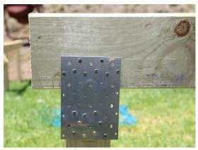
Complete filling the footing holes up with concrete and after a minimum of four hours add hardware. Brace & anchor piles: 160x110x1mm s/steel Nailon plate with 8-30x3.15mm s/steel product nails into bearer & pile & 2-100x4mm s/steel skew nails (not shown)
