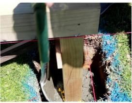
Begin filling holes with concrete taking care not to disturb the SubBases. When SubBase is covered rod the concrete with a rod or spade to ensure there are no air gaps under the SubBases.
