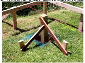
Plumb piles up in their correct location, fix temporary braces to the end piles in each line and attach to pegs set into the ground.
