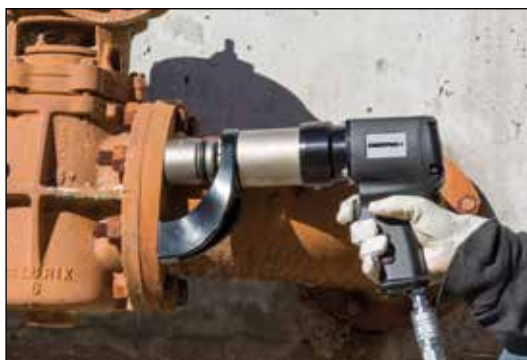
◀ The PTW1000 makes quick work of this flange maintenance job.
