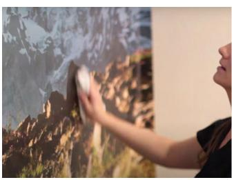
Apply the remaining panels using the same technique. Each panel has been printed with a 3 cm overlap and it can be double cut.
