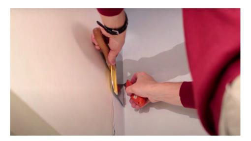
6. Finish off by trimming any excess material using fresh blade. Smooth the wall and remove any paste excess with sponge and clean cloth.
