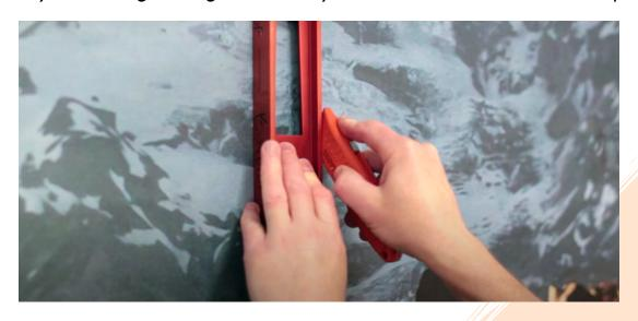
2. Carefully cut through both layers of the material. PLEASE NOTE to use very sharp blade, snap off the blade after cutting each panel. Make long cuts without lifting the blade.
