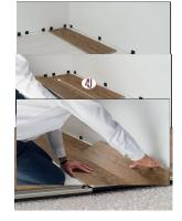
Figure 7: Continue alternating planks on rows 1 and 2. Ensure planks are properly aligned along the chalk line and against the spacers. Finish rows 1 and 2 in this manner, cutting planks at the end of the row as necessary. Ensure that the end planks are a minimum of 6" (150 mm) in length. If necessary, adjust the length of starter pieces to insure minimum plank lengths for each row, with proper end joint stagger row to row.
