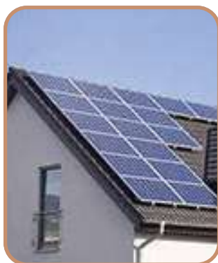
Home energy storage
