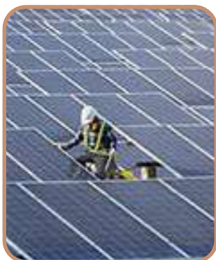
Solar energy storage
