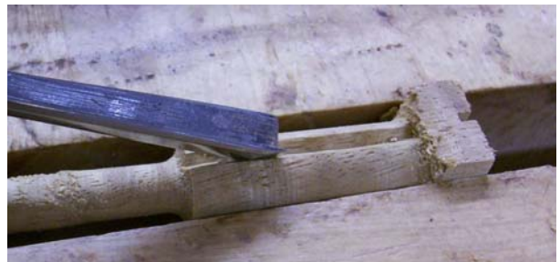
Figure 55 Cut groove in #43 with "V" chisel
