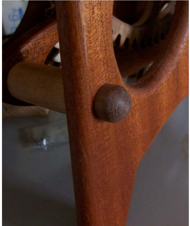
Figure 84 Nut cover # 37 glued onto hex nut
