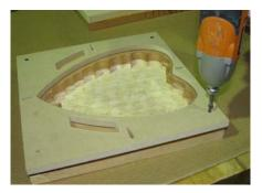
Install the template carefully by lining up the marks made previously. Mount the template securely using drywall type wood screws. Screw holes are provided but additional screws may be used if needed. Templates should be secure and screw heads countersunk in to the template. Be careful to place screws into the material in areas that will be cut off later.
