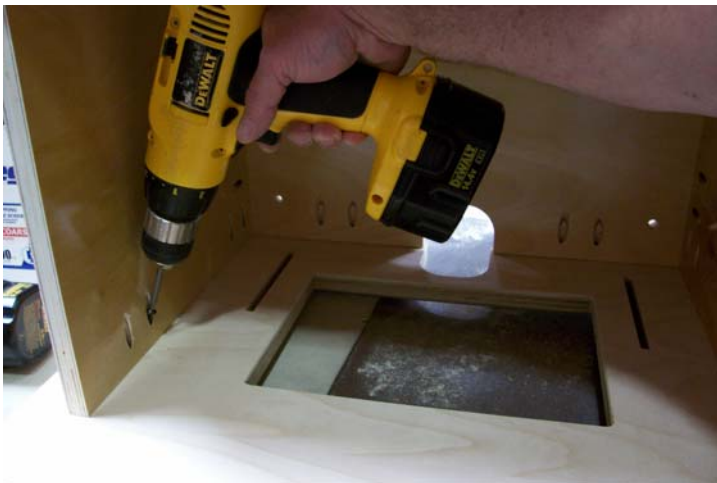
Place screws in all 12 holes that secure top to base.
