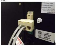
6. Plug the remote sensor cables into the splitter device at the Wine Guardian unit along with the communication cable for the remote interface controller. (Fig. 5)
