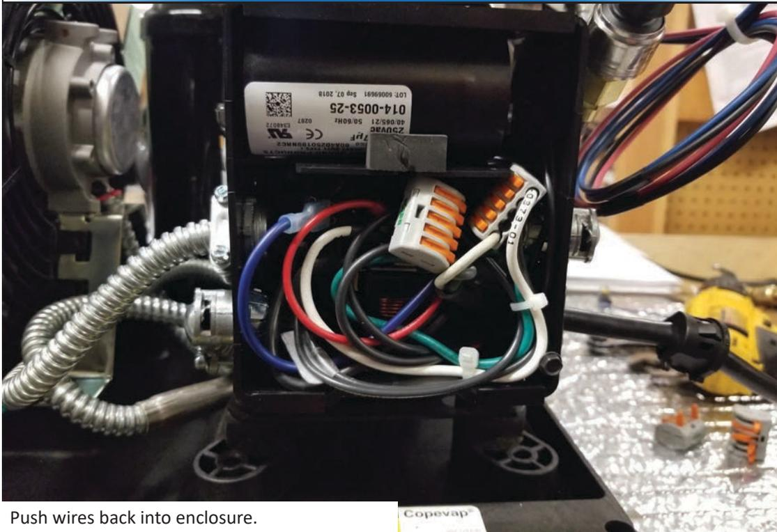
Push wires back into enclosure.
