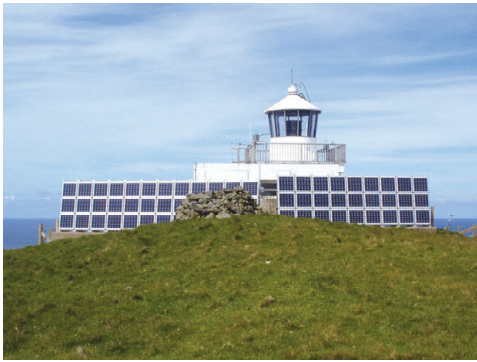
Plate 9. Lighthouse on Toa Rona powered by solar panels that have replaced the previously polluting diesel engines. The ancient summit cairn in the foreground is nesting habitat for Leach's Petrels, 18 June 2016. © Stuart Murray
