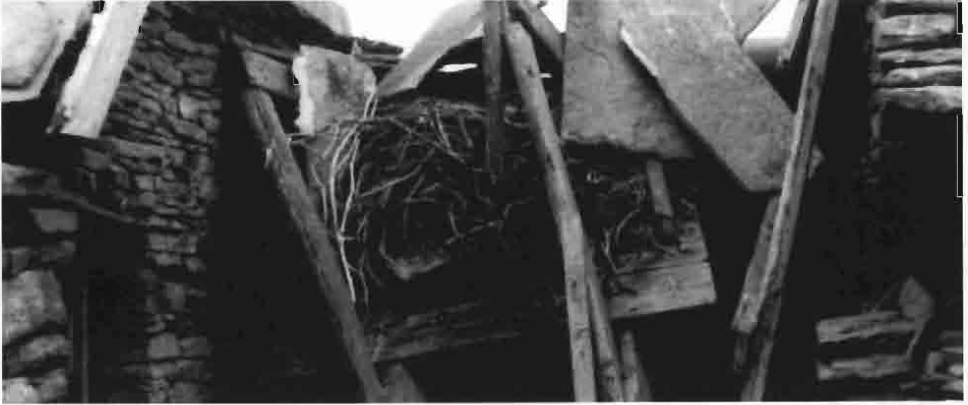
Common Raven nest on collapsed roof beams and stone slabs
