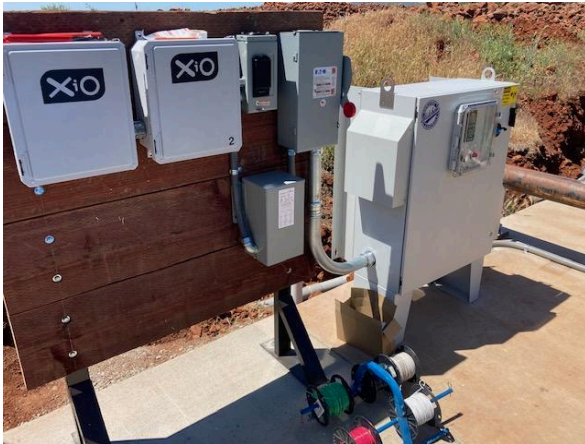
Figure 3. FIU and Modem mounting example
