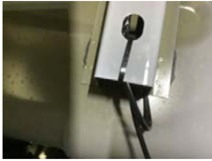
23. Connect wires and cable tie in place
