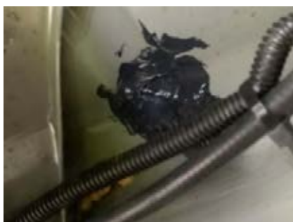
32. Cable tie the wires from the back and the power loom to the hand brake cable
