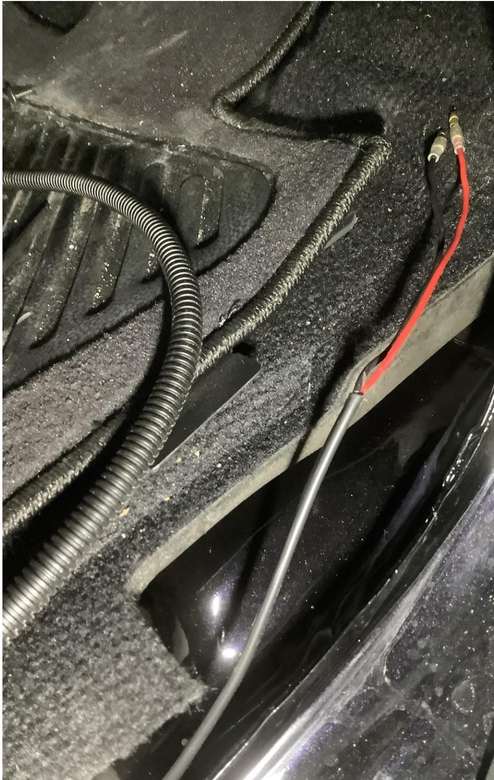
Connect power cable to battery and bring into cabin through the rubber grommet behind the glove box and then over to the drivers footwell area
