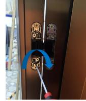
Conversely, turning the screws counterclockwise will move the door horizontally in the opposite direction.
