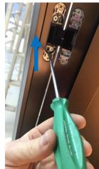
${\it 3. Tighten the loosened screws. Repeat this process for the other hinges.}\\$
