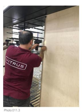
Place the Decorative Back Panel - Middle, one of the interior wall finish panels, into its designated location, ensuring proper alignment.
