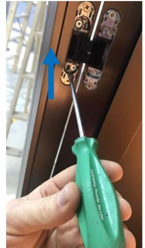
3. Tighten the loosened screws. Repeat this process for the other hinges.
