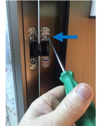
1. Use an allen key to loosen the two screws (indicated in the photos) on the cabinet body portion of each door hinge.
