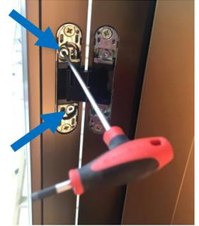
2. If the adjustment plate of the hinge is slid upward with a screwdriver, the door moves upward. Likewise, the door moves downward if the adjustment plate is slid downward.
