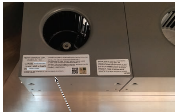
Rating label location
