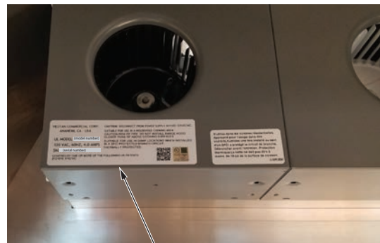
Rating label location
