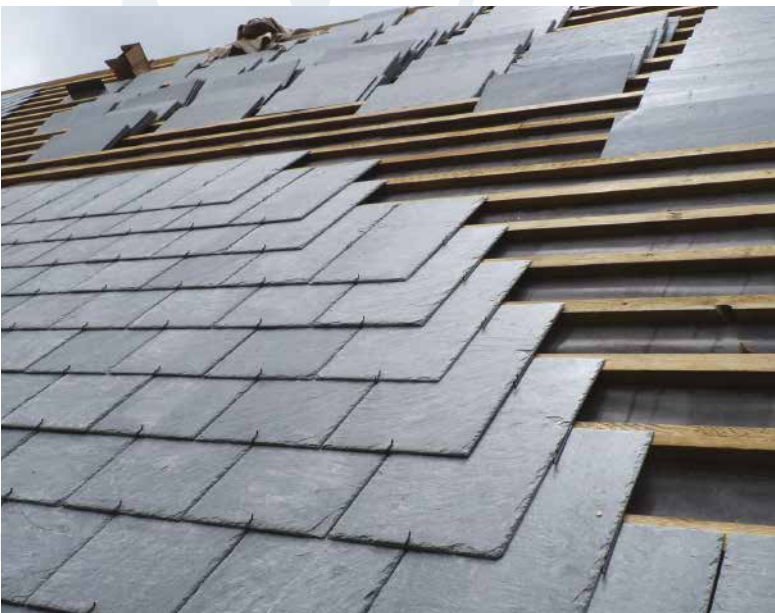
Slates graded and sorted into batches of equal thickness prior to installation
