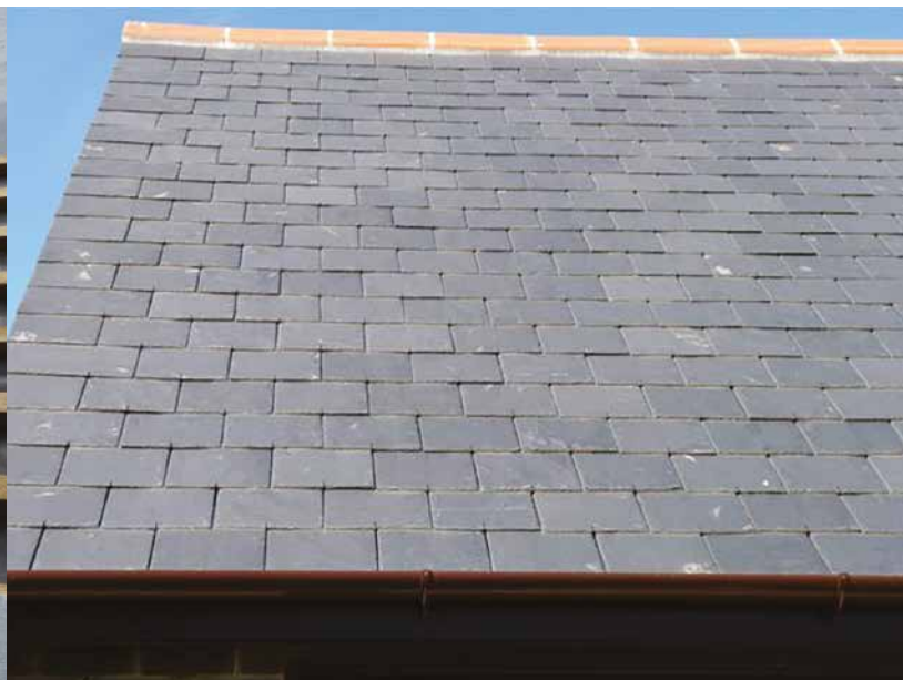
The result of installing slates without prior grading, slates of varying thickness in the same course, an unsightly, "gappy" roof slope!
