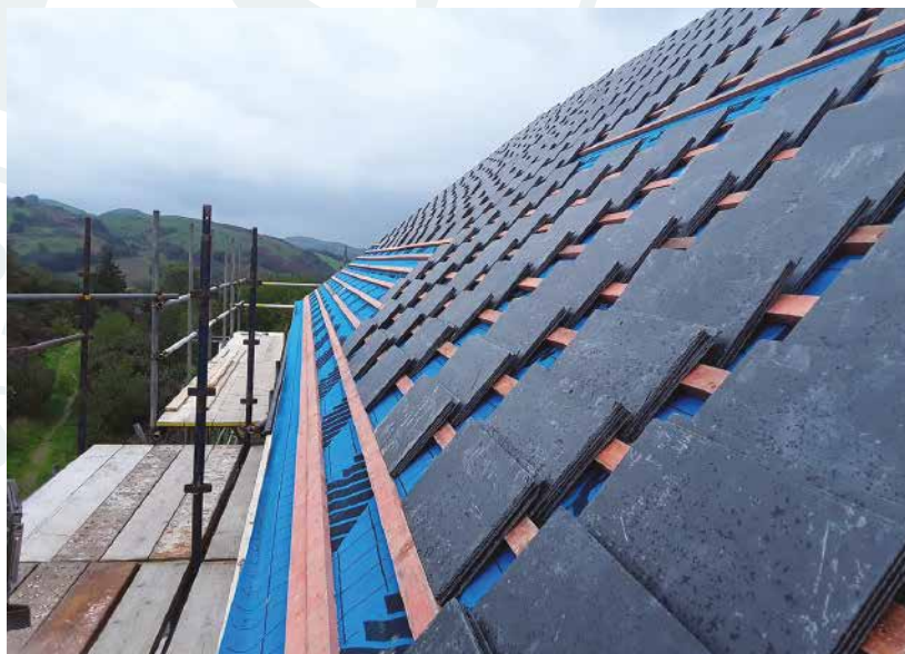
Use of chalk line to mark, perpends, half bond and slate head-line.
