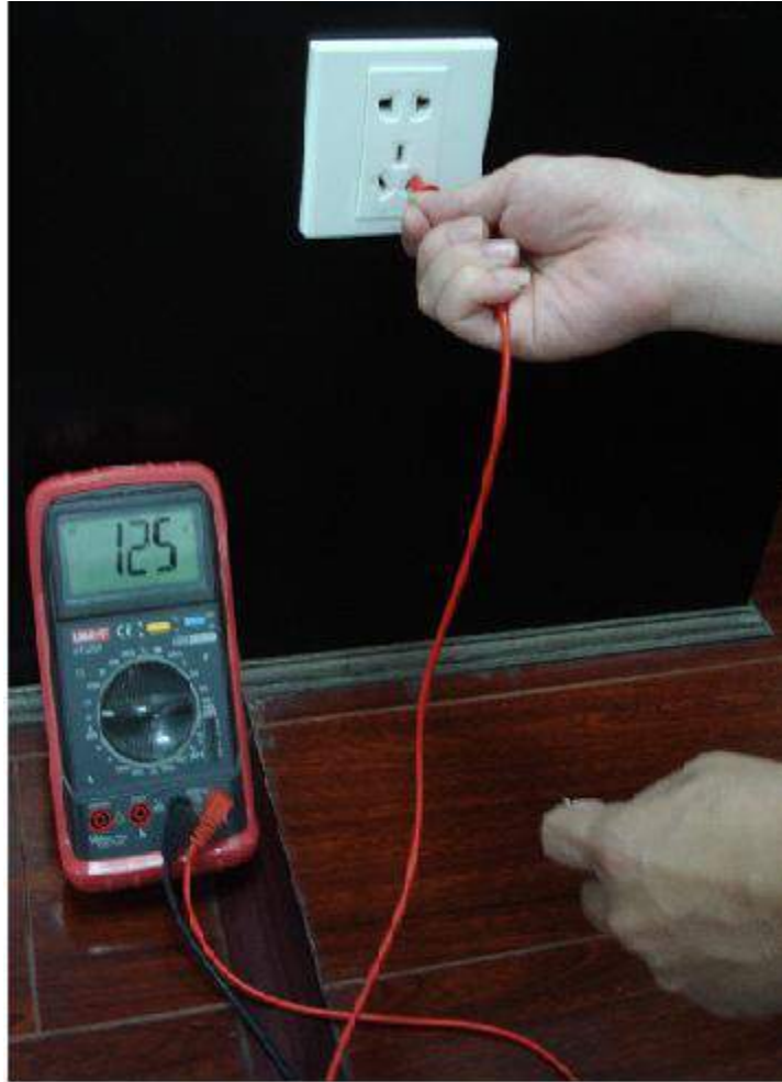
Appendix Figure 7-6 Check live cable connection
