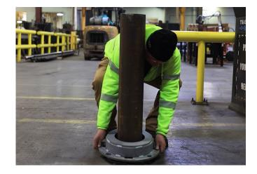
**Step #6:** : Drill down the nuts over the anchor bolts to lock the system into place, making sure the Plate is flush with the ground.
