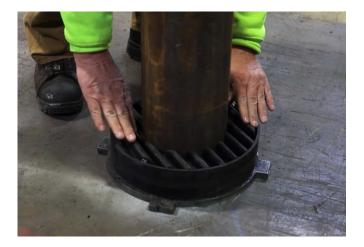
**Step #5:** Carefully slide the gray Base Plate Cover over the top of the Steel Bollard, using the side handles. Ensure the System Base Plate holes are lined up with anchor bolts.
