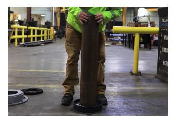
**Step #4:** Slide the Rubber Flex Topper over the top of the Steel Bollard and press into the Rubber Flex Base, making sure it's level.
