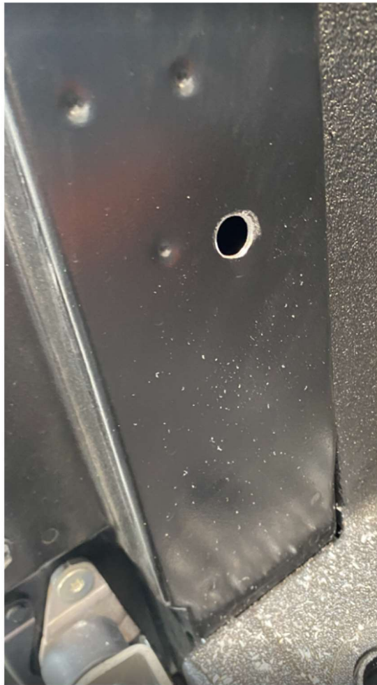
Figure 5: Correct hole drilled.
