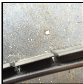
... center steel rib of the strip. You will make two vertical cuts approximately 1/2" from the centerline of the planned hole
