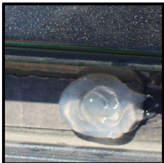
Next apply silicone over the holes
