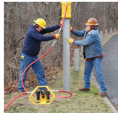
Additional Filter-Regulator - Lubricator recommended with the PD-200G increases tool-life.
