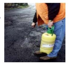
Bondade® is easy to apply and requires no special equipment. Simply sweep debris and water out of the repair area, spray Bondade®, and then patch using your regular cold or hot asphalt mix. Unlike other bonding agents, Bondade® can be applied to damp surfaces.
