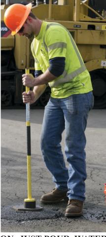
SIMPLE INSTALLATION: JUST POUR, WATER AND TAMP FOR A PERMANENT REPAIR.
