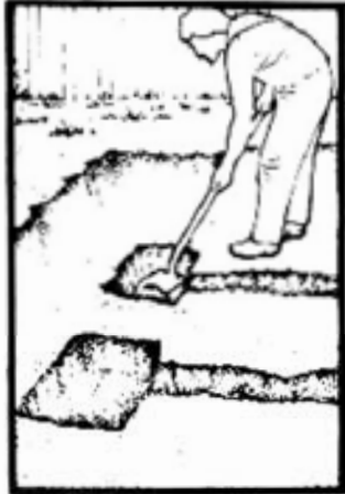
18. Excavation trenches for the base channel 76mm wide x 76mm deep.
