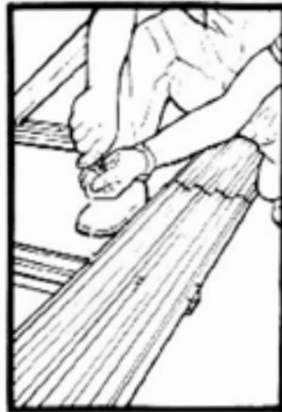
20. After excavations are complete, assemble the pressure plates to the pool frame constructions. Using the 4 self tapping screws (3) attach the pressure plate (17) to the base channels (16). Using the bolt 24 connect pressure plates together. Tighten with washer (26) and nuts (25).
