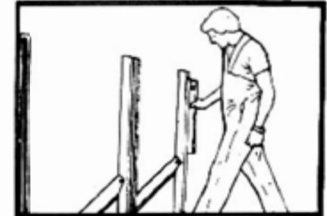
23. Check whether all uprights are level, in line, and level with each other.
