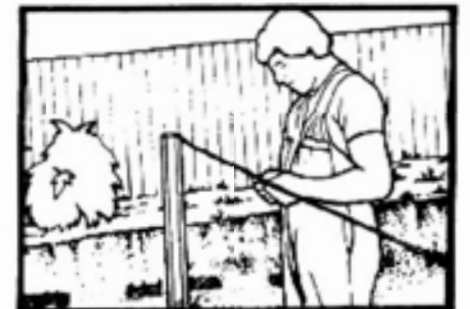
25. Use a line level to check levels across pool to opposite frames.
