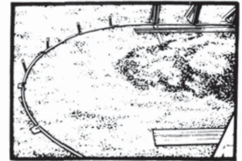
37. Slide the end rails into the connectors leaving approximately 32mm gap between them, and position with stakes so the rails conform to the radii marked out previously.
