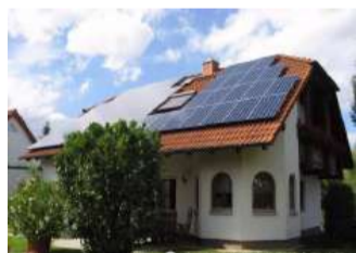
Home energy storage
