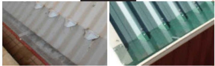
Corrugated Roof Saddle on every second rib
