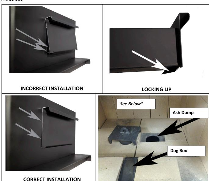
\*DAILY --Inspect the firebox for ash accumulation; remove excess ash and follow instructions in your owner's manual regarding disposal. Ash should not be allowed to accumulate in the stove to the point that it covers the dog box hole. The ash dump plug in the firebox may be removed and ashes raked into the ash pan below for temporary storage. Remember to replace the ash dump plug.
