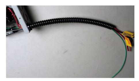
Run all five wires through the conduit tubing.
