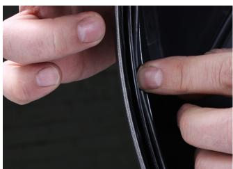
**Step 9:** Fit wires into pre-existing groove channels and run them down to the drilled hole.
