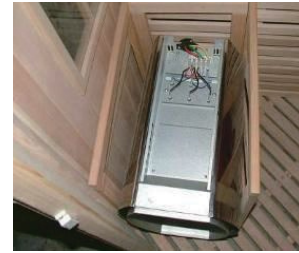
Connect the power supply line of the stove
