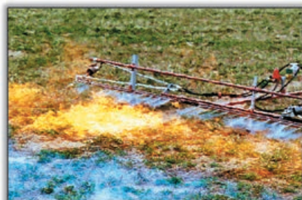
The Liquid Spray Process In Action!
