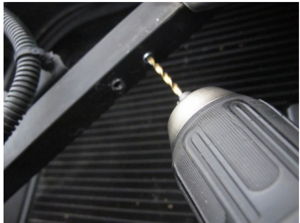
Fig. 7-E: Drill heat exchanger mounting holes
